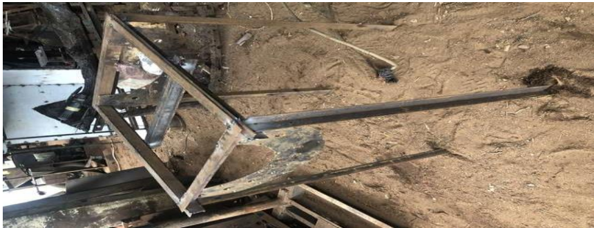
Figure 9: Frame under production
